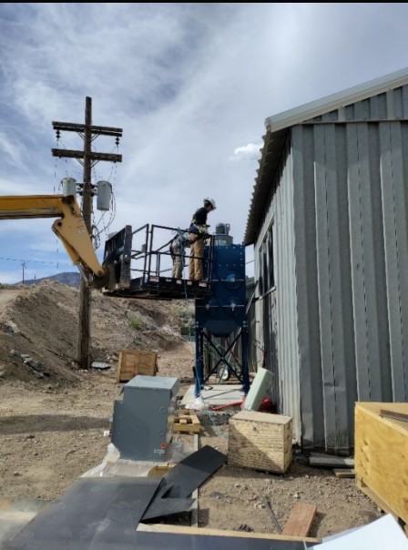
New baghouse installation
